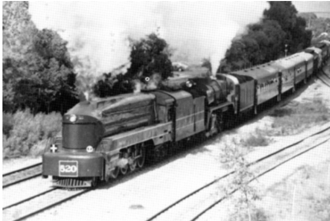
520 and R766 pass Salisbury enroute to the Barossa Valley on 8th June Photo: R. Platt
