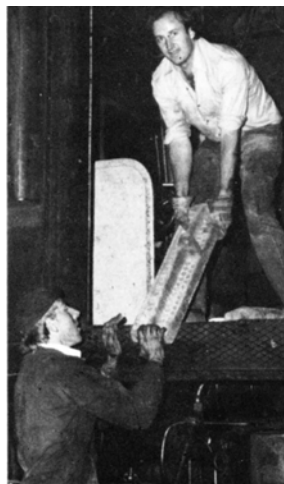
Volunteers at Dry Creek working on superheater elements (top) and installing heavy firegrates (below) Photos: Roger Currie
