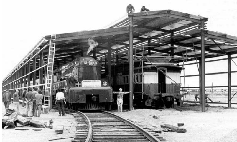
520 noses out of the depot shed on 21 Nov 79 whilst testing for clearances
