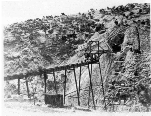
Sleeps Hill Viaduct in course of construction.
