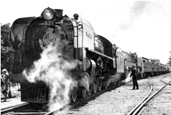
Engines 621 and 520 have just arrived at Victor Harbor with the 12 car inaugural Southern Encounter on 18th October 1986 following rehabilitation of the Strathalbyn to Victor Harbor railway. This was the first occasion when volunteer SteamRanger crews were used Photo: Roger Currie
