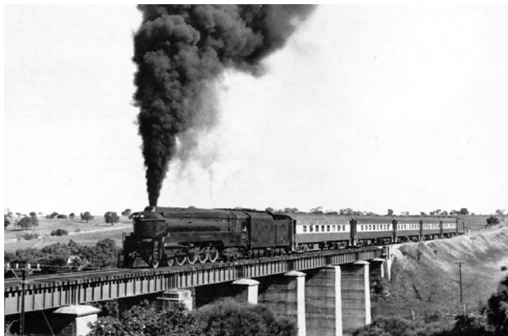
Loco 526 races across Currency Creek bridge with the up South Coast Limited special on 18 Oct 1969 Photo: Dean Harvey
