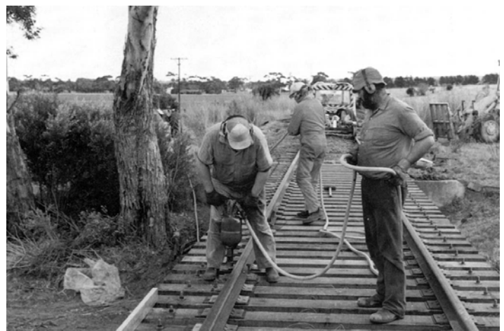
Butch Collett hard at work on the "dog knocker" at Swamp Creek bridge on 30th April 1991 Photo: Dean Harvey
