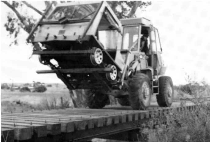
A novel way to transport a section car over Black Swamp bridge when the rails were removed for bridge retimbering. Photo: Dean Harvey
