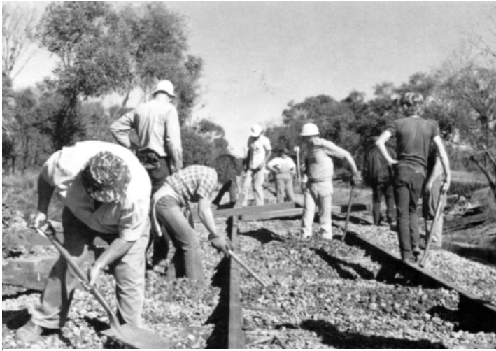
Resleepering at the 100km mark near Black Swamp in the Strathalbyn to Victor Harbor CEP upgrading project in 1986-87. At one stage there were 96 people on the payroll in this project, whereas in the 1900-91 project between Mt Barker Junction and Strathalbyn the maximum was eight workers and then only for a short time. Photo: Dean Harvey
