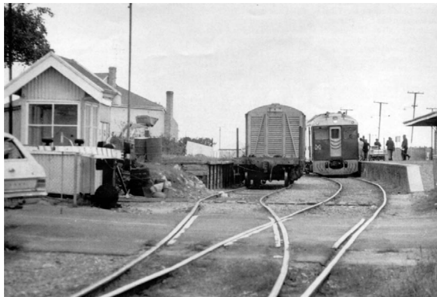
Bluebird 250 the class leader, at Pt Elliot with the up morning passenger run in May 1969. As only one SAR officer was on duty at Pt Elliot it was normal practice to lower the gates before arrival of the railcar and then return to the station to attend to passengers and goods. The short boom gates were usually set against road traffic for 5 - 10 minutes, a source of irritation to many locals, who often overcame the delay by zig zagging around the gates to negotiate the crossing. One such vehicle is seen disappearing to the left. The boom gates and gate kiosk were removed shortly afterwards and the siding was terminated on the other side of the road crossing. Photo: David Worth
