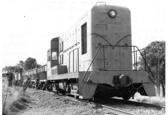
SteamRanger Z class hopper wagons and ballast plough hauled by DE engine 351 running ballast near Gemmels in October 1990 during the major track upgrading project Photo: Roger Currie
