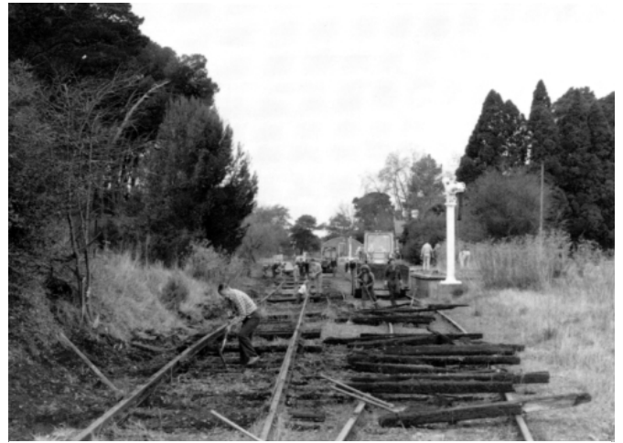
Volunteers replacing sleepers on No1 Goods Siding at Mount Barker in 1986. This siding is a loop and is used to run engines round a consist when trains terminate here. The poor quality of the sleepers already removed can be observed Photo: Dean Harvey
