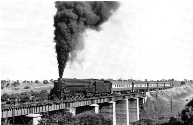
Engine 526 races across Currency Creek bridge with an up South Coast Limited special 18 Oct 1969
