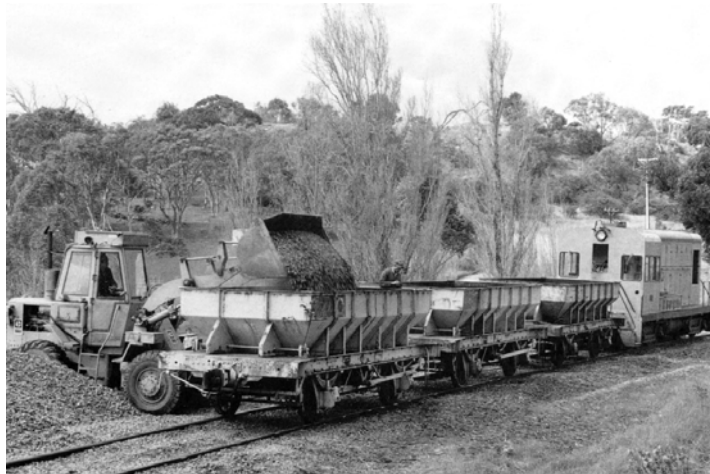
After running one train load of ballast DE351 pauses at Gemmels so that three of the SteamRanger Z class hopper wagons can be reloaded Photo: Roger Currie
