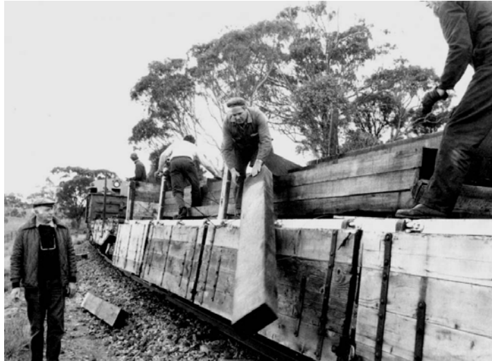
Volunteers Philip Neville and Kim Critchley unload sleepers at positions indicated by Dean Harvey (walking alongside) near Gemmels on 15 July 1990 Photo: Andrew Gramp
