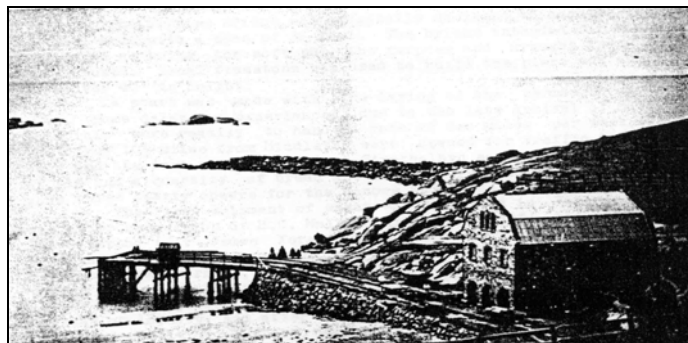
A view of the foreshore at Pt Elliot (circa 1854 - 1864) showing tramway tracks, trucks, jetty and Government store
